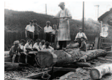
Two men one above and one below planking an oak tree in a saw pit.
