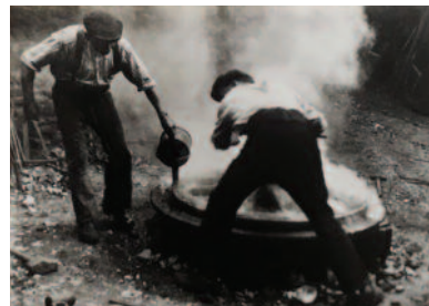
Blacksmiths Mark and Harold Fletcher hooping a wheel with a hot metal rim. The metal rims were heated up and quickly cooled with water to shrink it on to the wheel.
